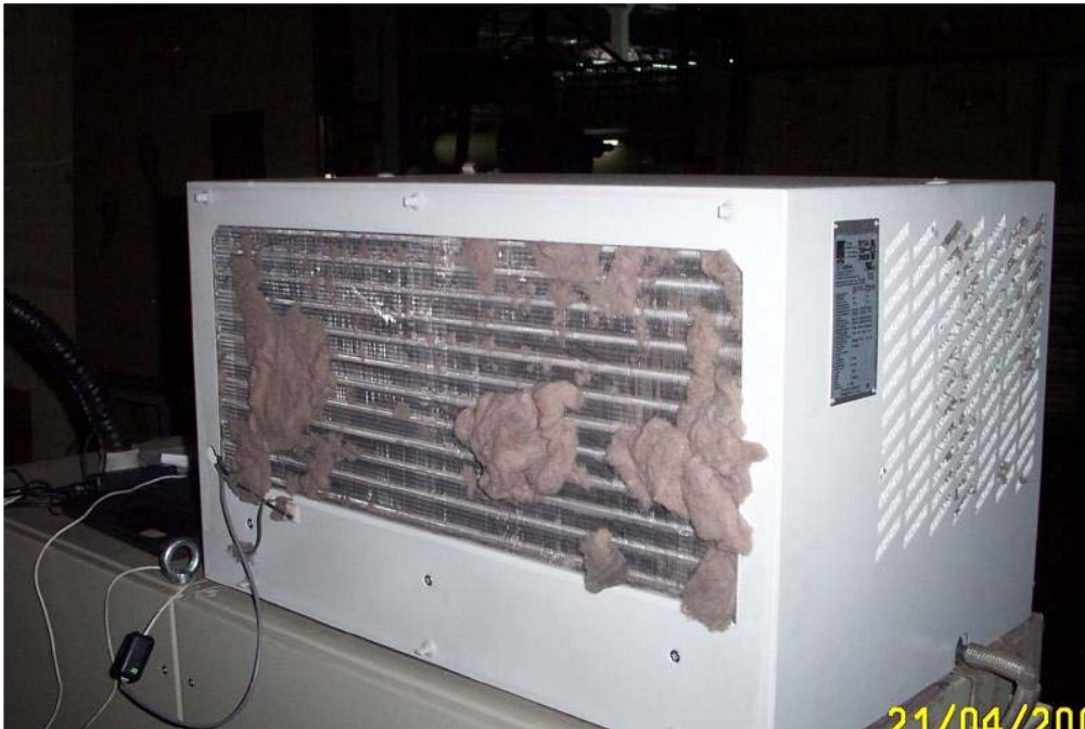
Heat exchanger without coating in textile industry
