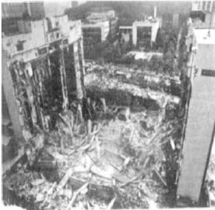
Sampoog Department Collaps, Korea 1995
